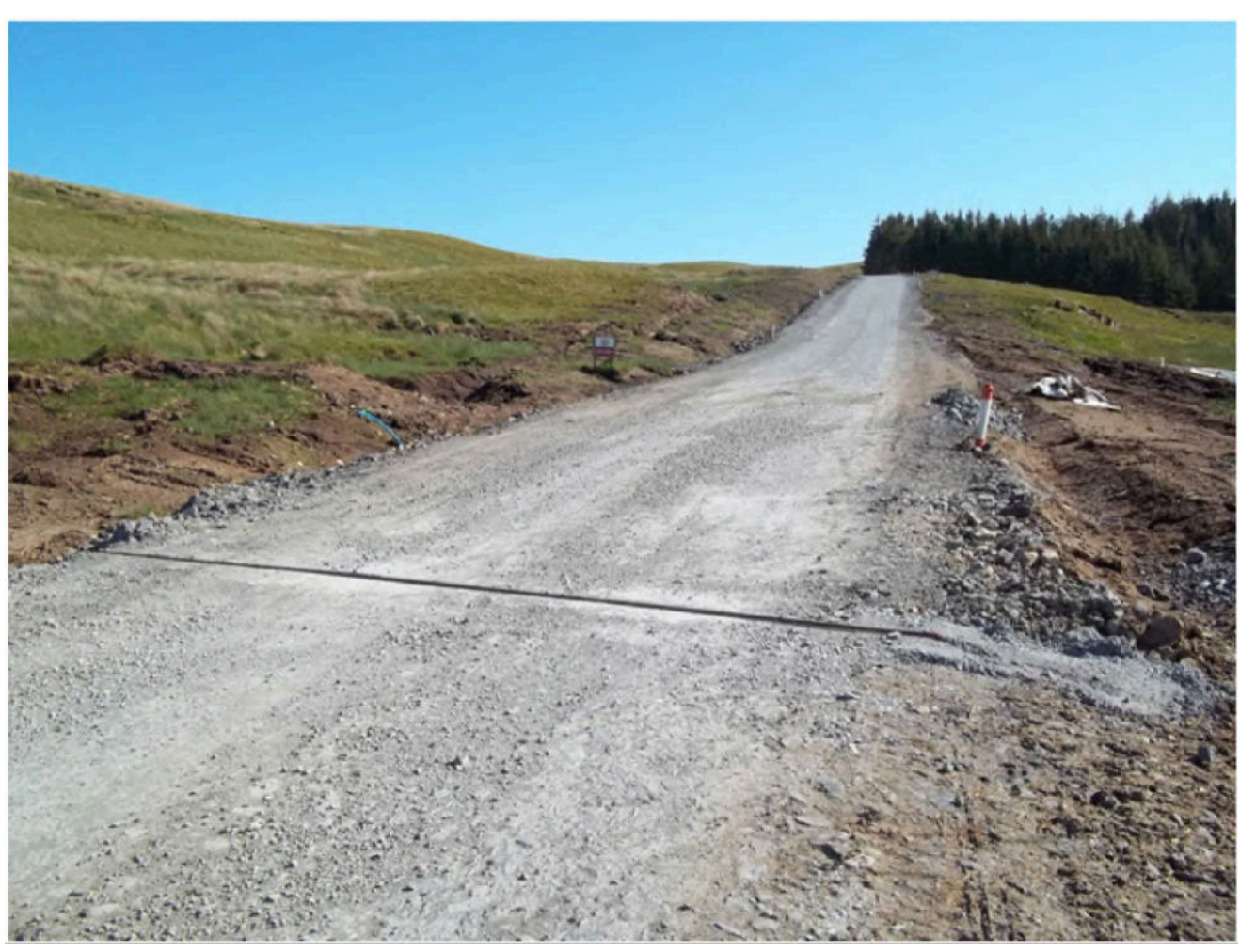
EXAMPLE OF ROAD GRIP INSTALLATION NTS
